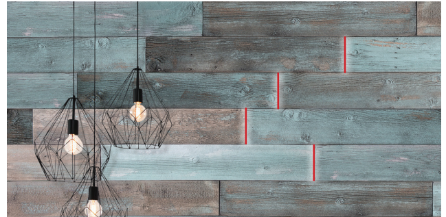
Example of staggered planks.
